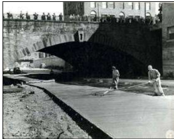
Paving of the conduit top where a highway would eventually run, 1945
