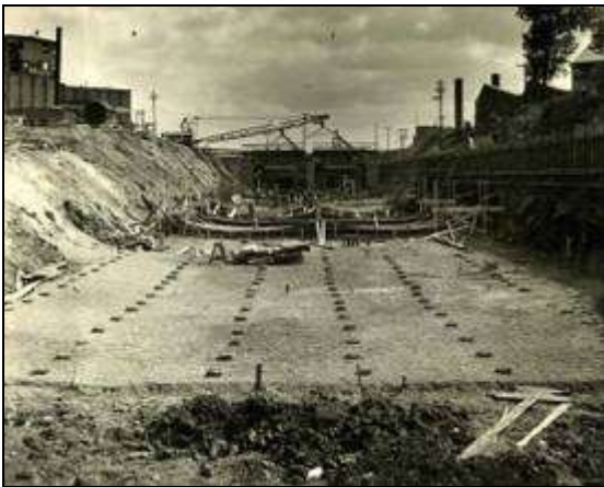
Construction on the first phase, 1941
