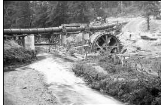
1916. The pipe temporarily carried cross-flow.
