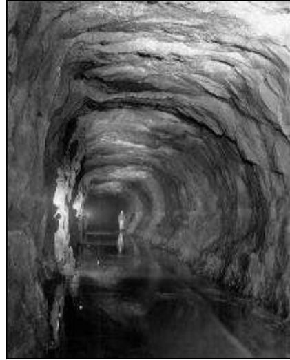
Tunnel yet to be concrete lined
