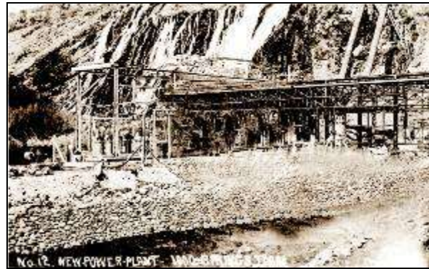
Powerhouse Construction, 1912. Note the twin spillways on the right.
