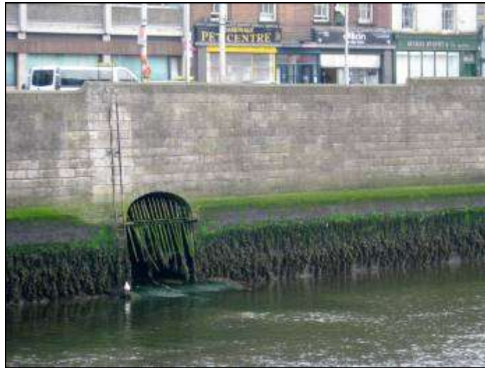
The confluence of the River Poddle and the River Liffey, visible at low tide through a grate in the Liffey walls.
