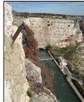
Looking upstream from the aqueduct
