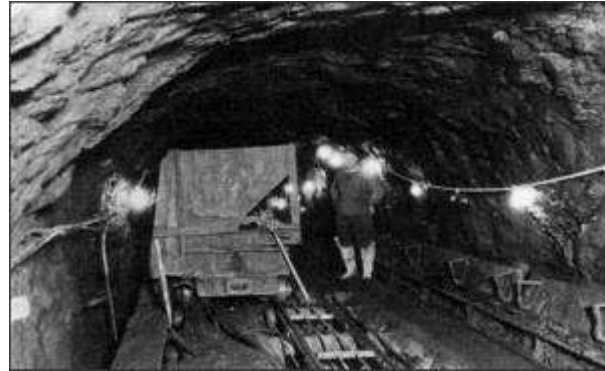
Construction prior to concrete lining.
