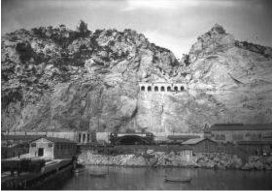
Above, photos from 1913. Note the cofferdam at the tunnel mouth and the multi-arched structure along the cliff above. We'll return to it later. The second photo documents an official visit.
