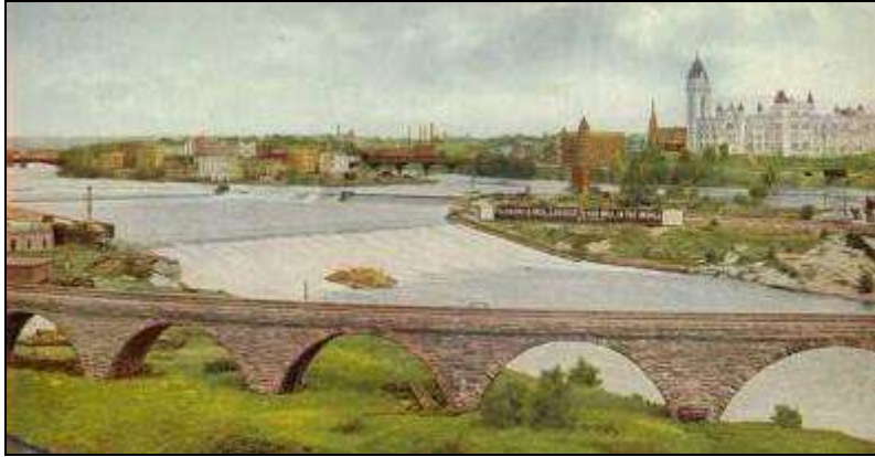
Underground River Plugged and the Mills Saved
