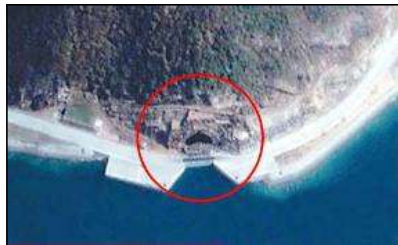
Completed Tunnel Entrance
