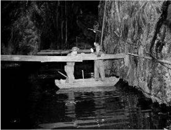
Nova Scotia's Malagash salt mine was opened after brine was discovered in a water well and mined until 1956. The photo is from 1944.
